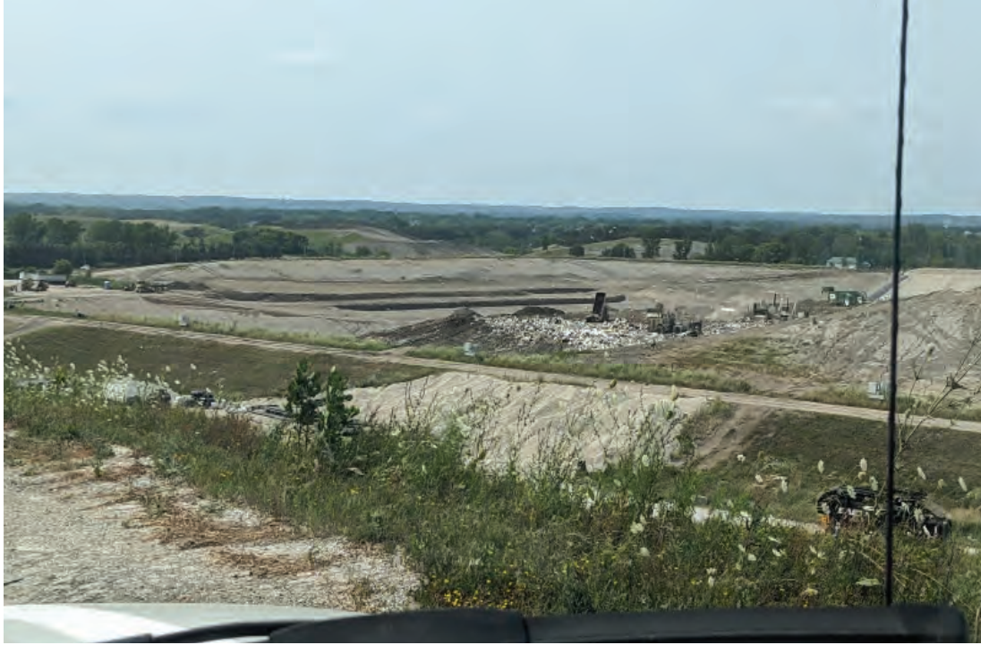
Terraced excavation of future cell
