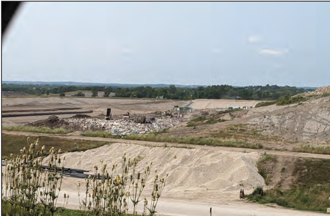
Phase 3 viewed at grade
